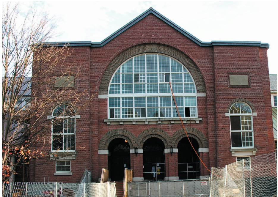
Modern techniques, like seismic Cone Penetration Tests, now allowed under the International Building Code, saved $50,000 - $100,000 in construction costs at the Dartmouth College Alumni Gymnasium in Hanover, New Hampshire.
