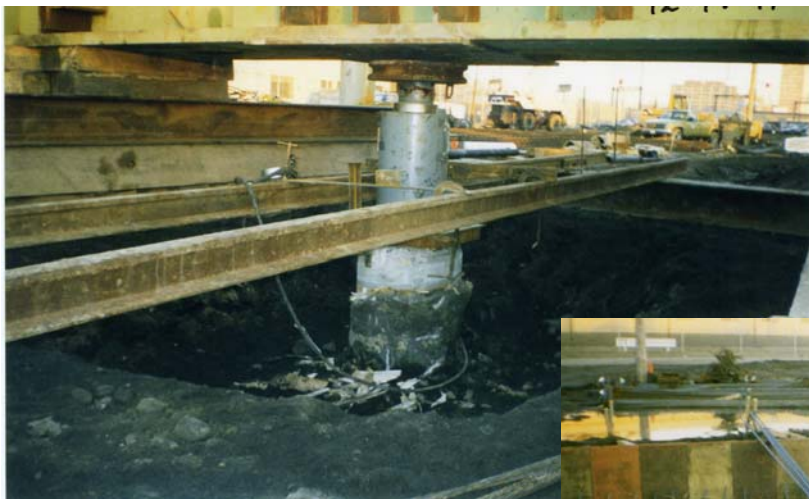
Load testing a drilled shaft
