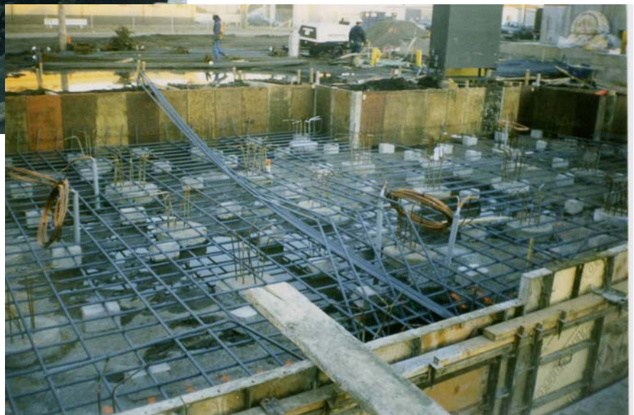
Preparation of foundations
