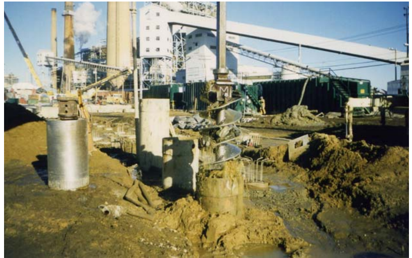
Drilled shaft being installed
